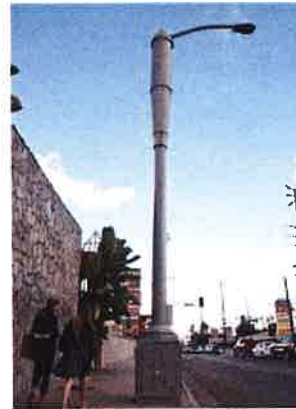
Effective small cell, light pole combination with equipment concealed in the base of the pole, except that new poles and equipment shall meet color requirement.
