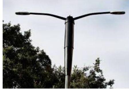
Sample small cell, light pole combination.
