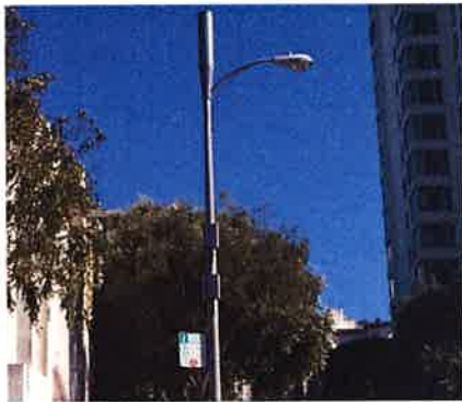
Effective small cell, light pole combination except that new poles and equipment shall meet color requirement.
