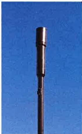
Acceptable tapered transition.
