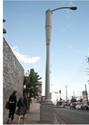
Effective small cell, light pole combination with equipment concealed in the base of the pole, except that new poles and equipment shall meet color requirement.
