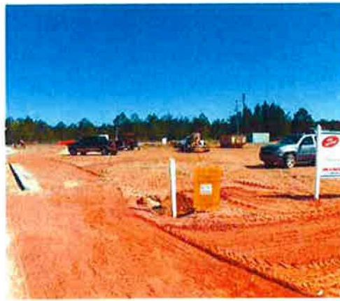
Proposed Bldg. 2 site
